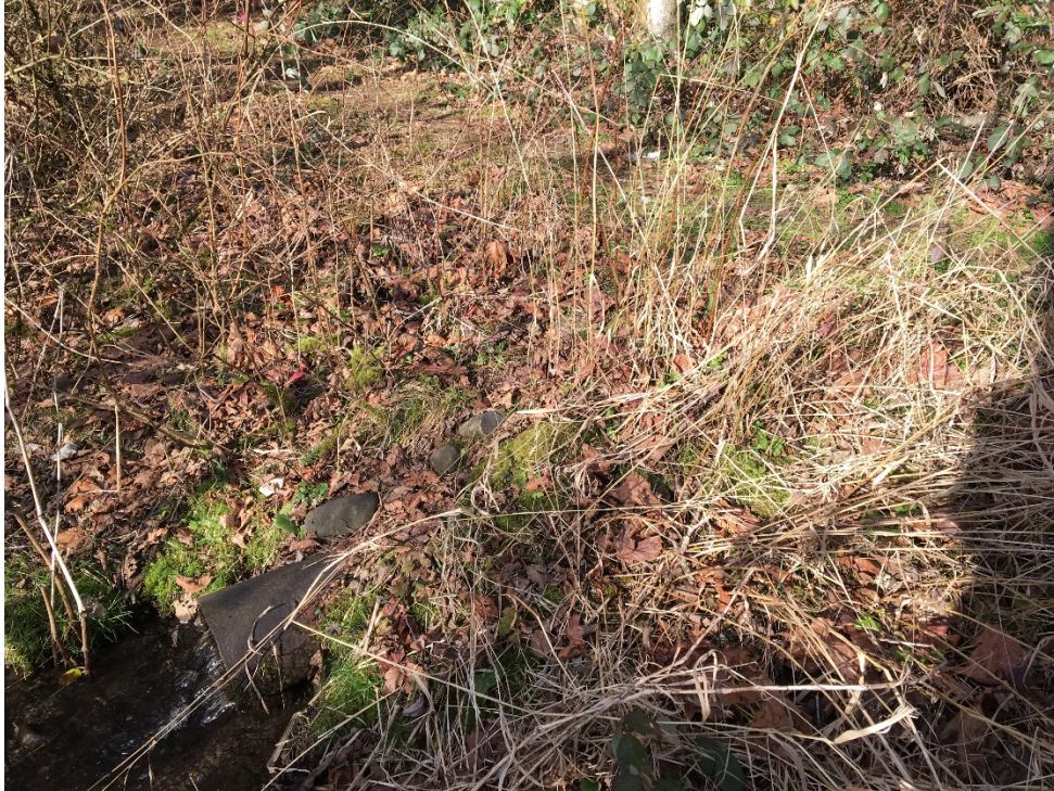
Photograph 4: Culvert outfall (bottom left) from East wetland at the abandoned access road crossing, where boardwalk proposed. Photograph taken January 14, 2018.
