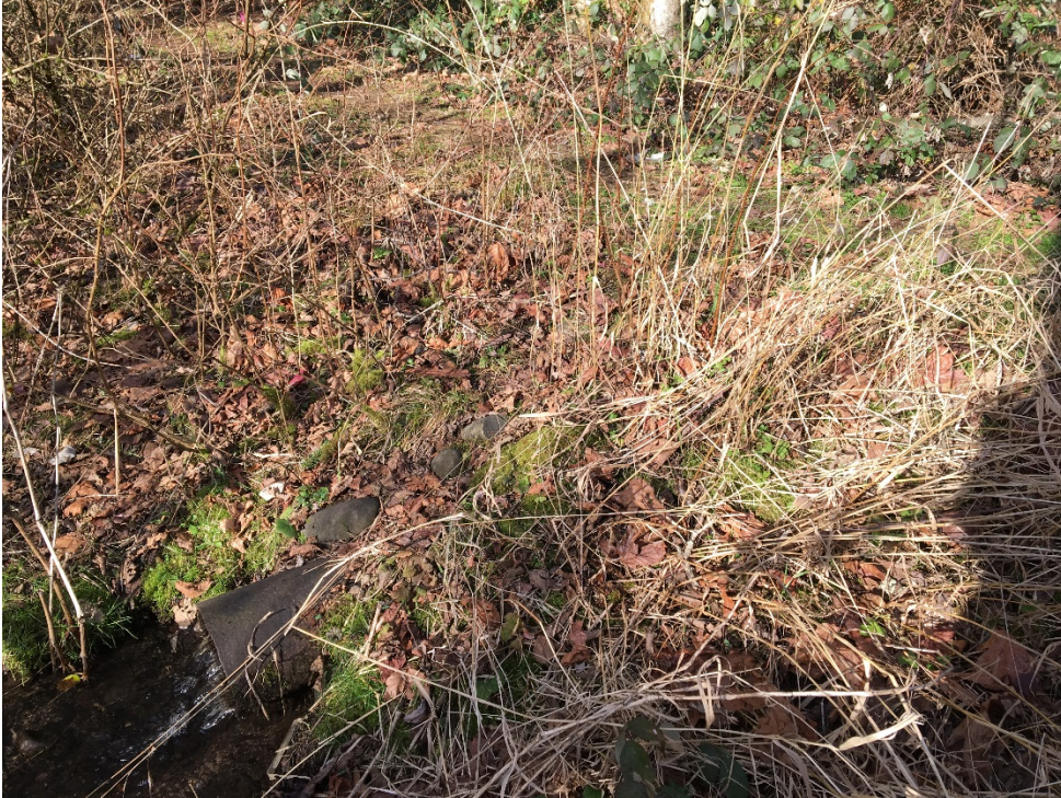
Photograph 4: Culvert outfall (bottom left) from East wetland at the abandoned access road crossing, where boardwalk proposed. Photograph taken January 14, 2018.
