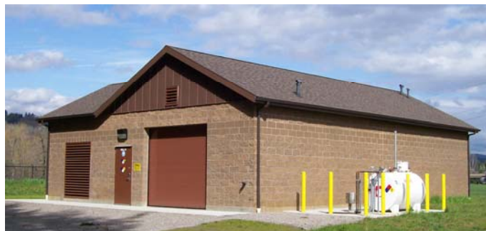
Well 14 Located just west of Goot Park, was completed in the summer of 2010.
