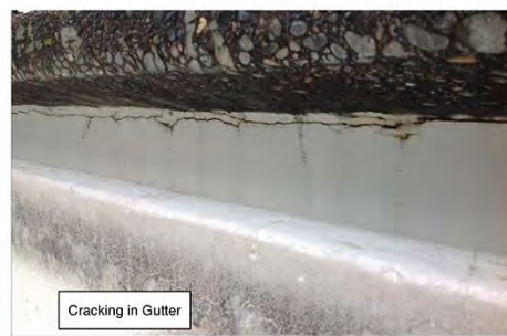
Insufficient Gutter Drop-Out
