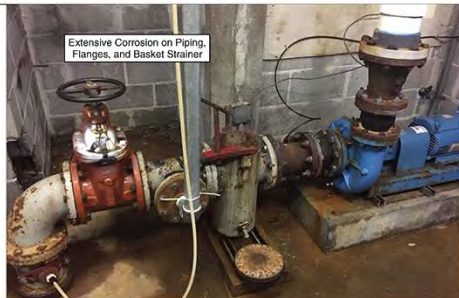
Extensive Corrosion on Filters
