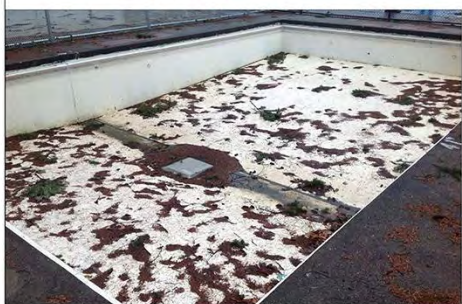
Deteriorating Pool Paint
