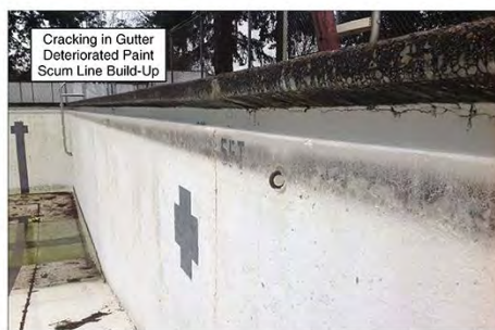
Cracking in Gutter
