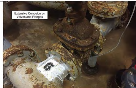
Paint Chipping, Peeling, and Flaking Away
