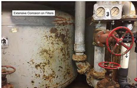
Extensive Corrosion on Valves Metal Piping in Pool System
