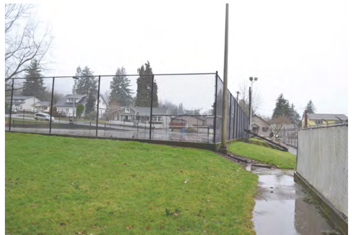
Exterior fence and foundation of tennis courts
