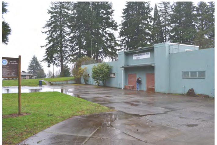
Pool facility entrance to restrooms and changing areas
