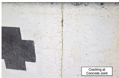
Deteriorating Pool Paint
