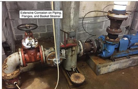
Extensive Corrosion on Filters
