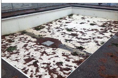
Deteriorating Pool Paint
