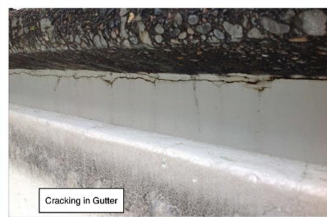
Insufficient Gutter Drop-Out
