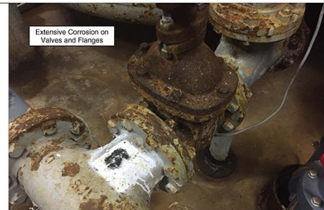
Paint Chipping, Peeling, and Flaking Away
