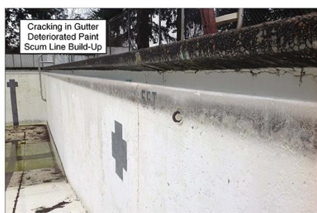
Cracking in Gutter
