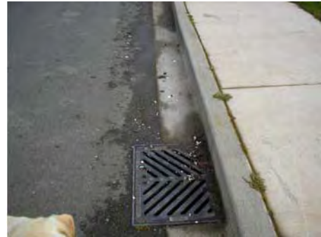
Latex paint residue on catch basin
